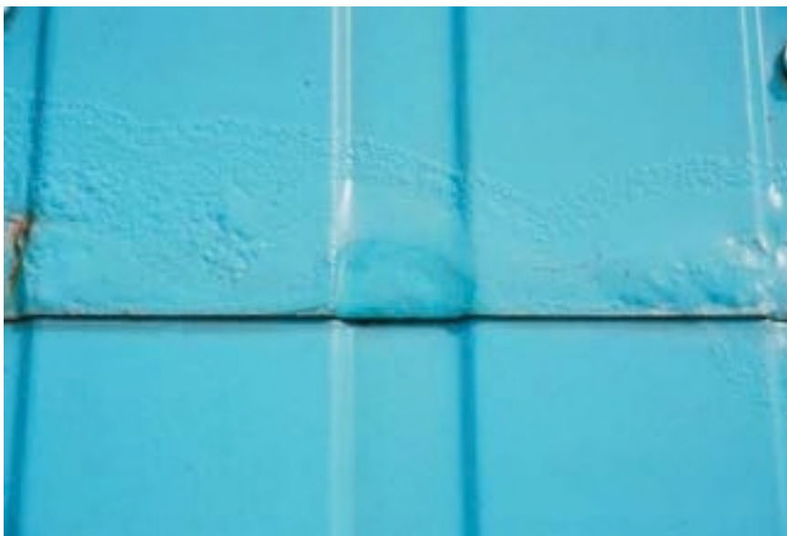
Figure 25. Paint blistering on a prepainted GALVALUME ® roof caused by poor end lap sealing.
