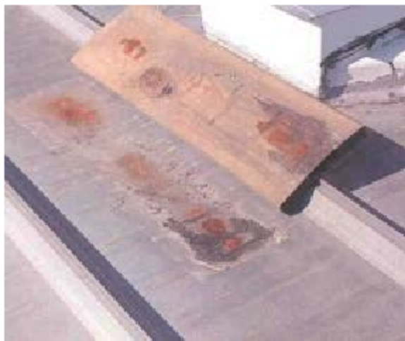
Figure 31. Corrosion occurred under the treated lumber because chemicals, particularly copper compounds, leached from the wood accelerating the corrosion.
