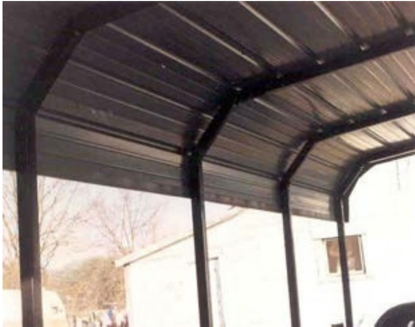
Figure 41. Improper roof profile design of a pole building with open sides does not allow rainwater to runoff along the curvature of the roof.
