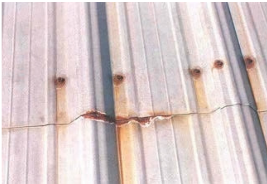
Figure 24. Crevice corrosion caused by poor end lap sealing on a GALVALUME ® roof.
