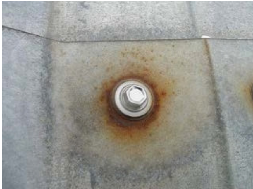
Figure 27. Photograph of red rusted metal filings on the surface of bare GALVALUME ® roof panel around a screw.
