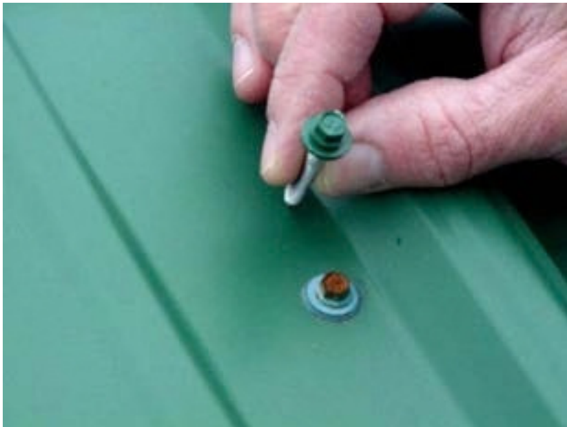
Figure 14. A close view of a non-matching screw with red rust and the correct screw, held in the hand, which should have been used for this application.
