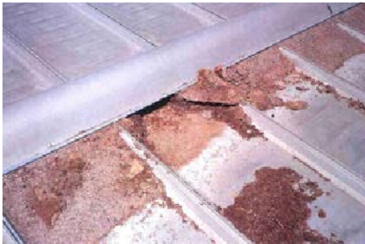
Figure 30. The wood chip debris piled near the ridge cap caused heavy corrosion of the roof panel due to water being retained by the debris.
