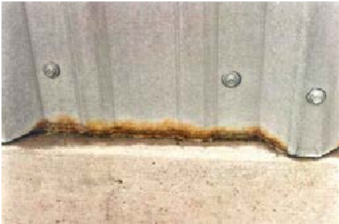
Figure 16. Premature corrosion at the bottom edges of the GALVALUME® panel caused by insulation wicking.
