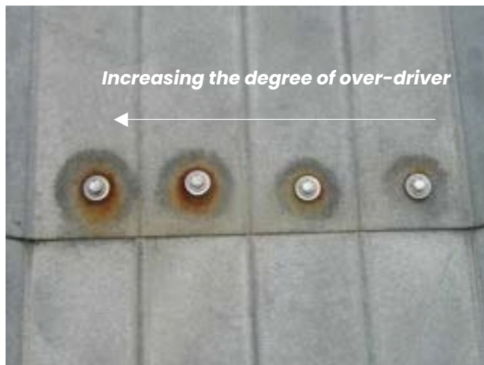
Figure 11. Photograph of the over-driven fasteners. The corroded area around the fastener increased with increasing depth of depression.
