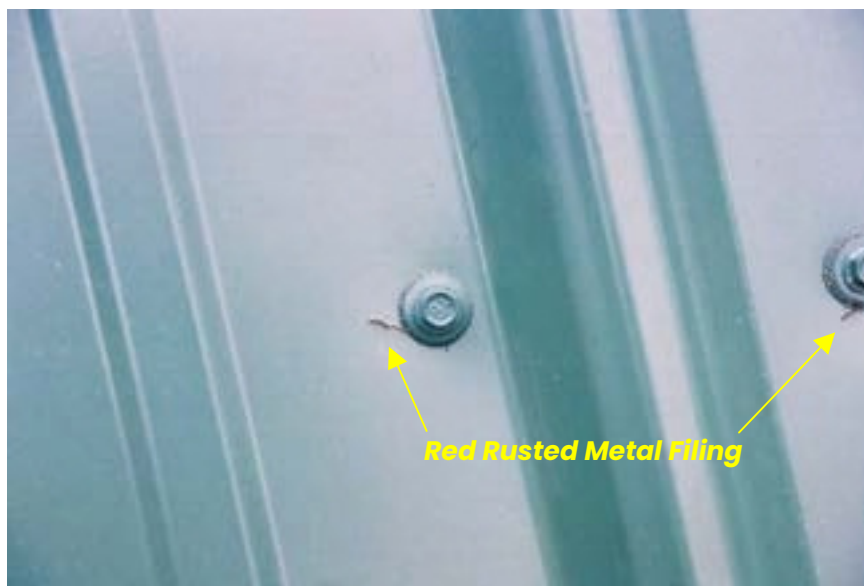
Figure 28. Photograph of red rusted metal filings from the screws on a prepainted GALVALUME ® roof panel.
