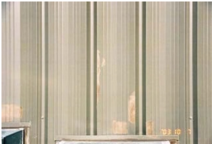
Figure 46. Differential chalking and fading appearance on prepainted hot-dip galvanized steel siding with improper touch-up paint.
