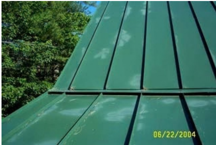
Figure 45. Differential chalking and fading appearance on the prepainted GALVALUME® steel roof with improper touch-up paint.
