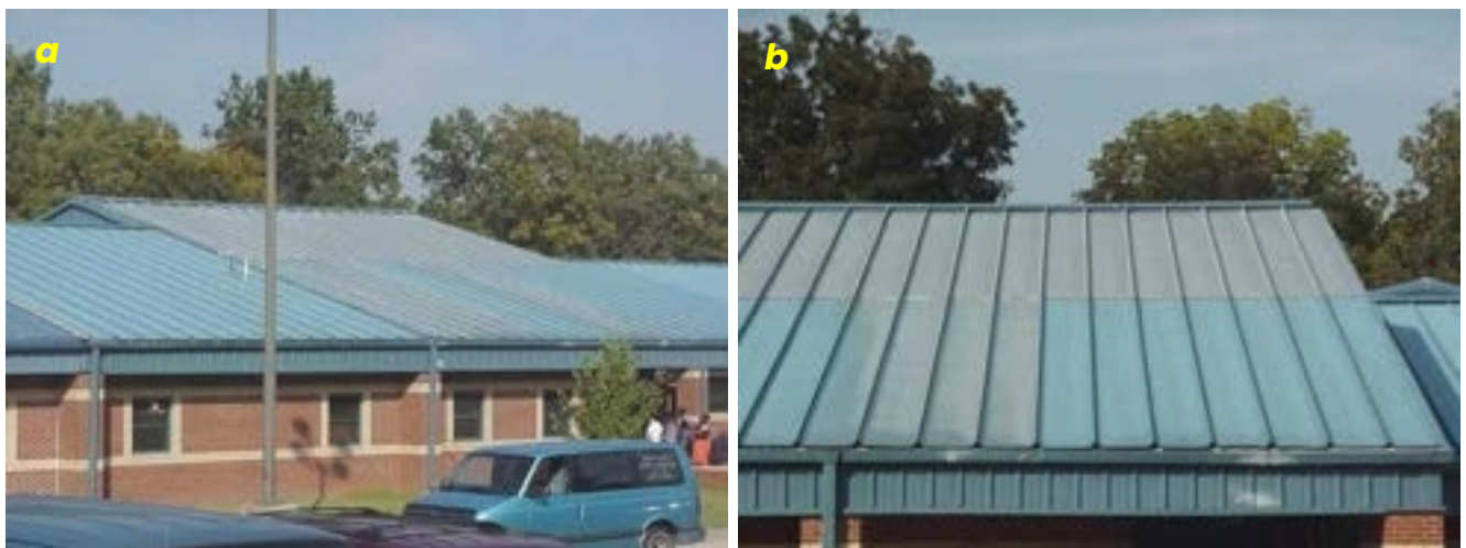
Figure 44. Non-uniform fading of a pre-painted roof with noticeable differences in color from one section to another section (a) and its close look (b).
