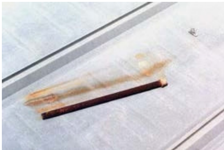
Figure 32. A piece of metal tube left on the roof caused staining and corrosion of the roof panel.
